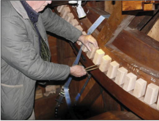
top: Checking the centres & spacing. right: Profiling the outer face.
